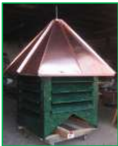
hoto of the new steeple which will be lifted and installed on the Chapel roof this week.
